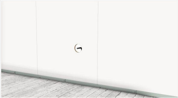
Make a hole at the desired position.
