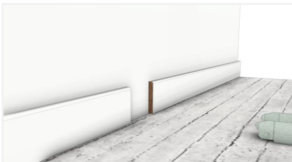
Make a recess in the skirting board the width of the wall.
