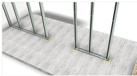
Now place the C-modules on the floor marking.
