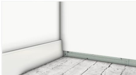
Let the click panel fit fully against the wall.
